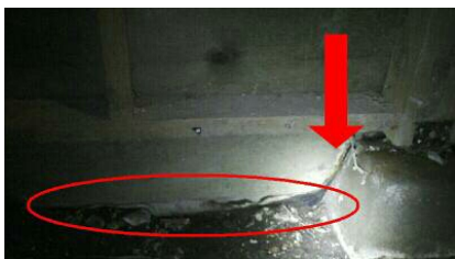
wood to soil contact
