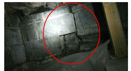
Southeast corner foundation
