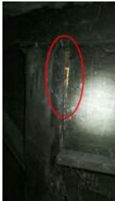
Gap in plywood skirting around base of home.
