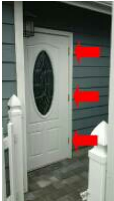
Patio door installed with hinges on exterior
