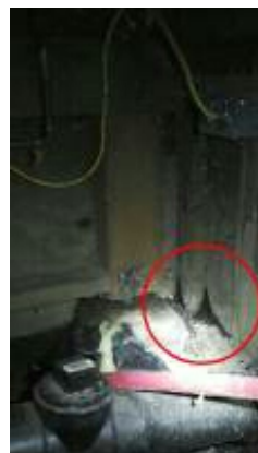
wood to soil contact
